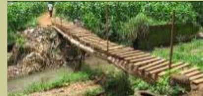
The initial bridge on the way to Mile 2
