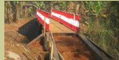
After the project a safer bridge with railings was in place
